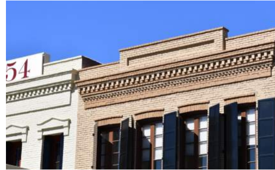
Flat parapets & masonry cladding
