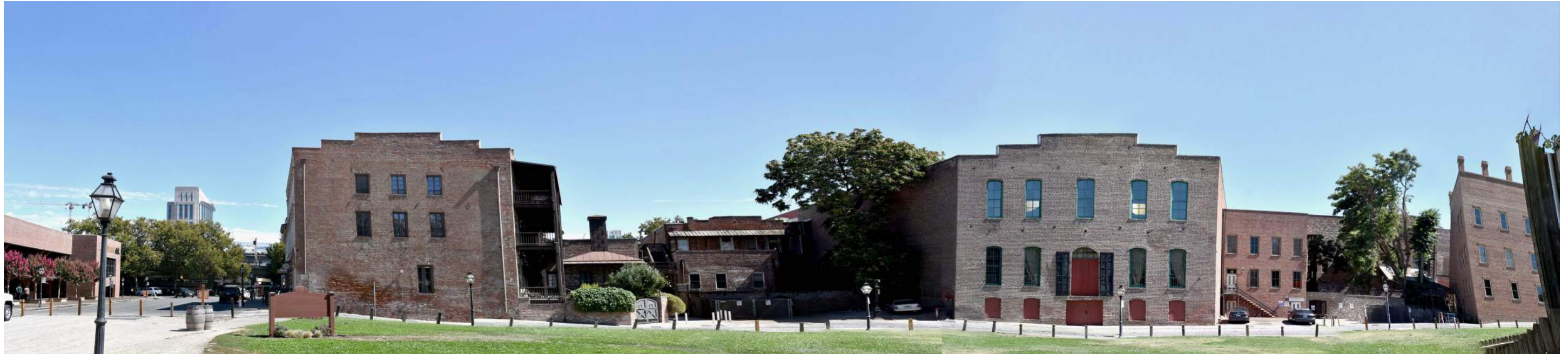
Elevation C: Alley elevation, looking east.
