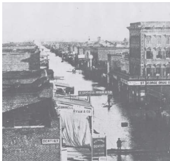
1861 J Street near Front Street
