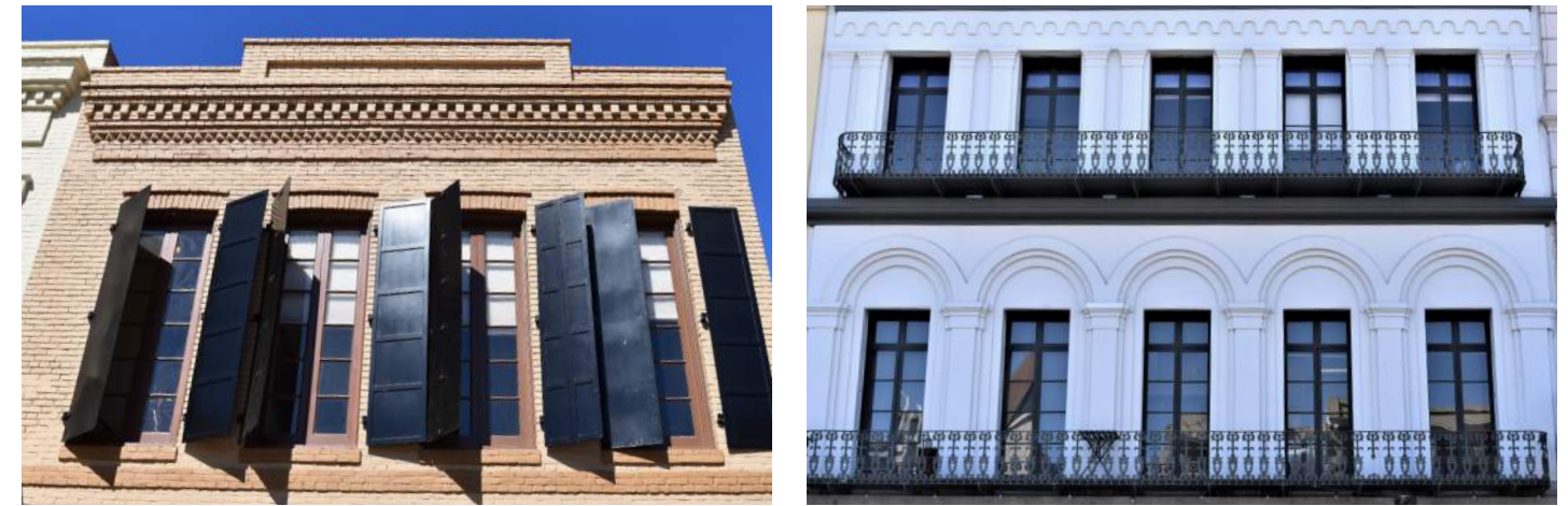
Figure 21: Windows and doors should be scaled and arranged to relate to the pattern of tall, vertically oriented, evenly spaced windows and doors at historic buildings.
