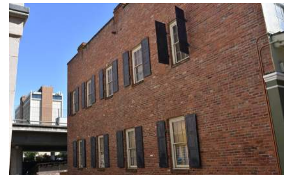
Brick secondary facades
